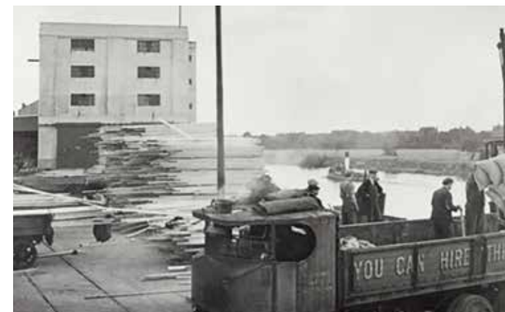
A large stack of timber on the wharf beside No.1 Warehouse in the 1930s (Canals & River Trust)
