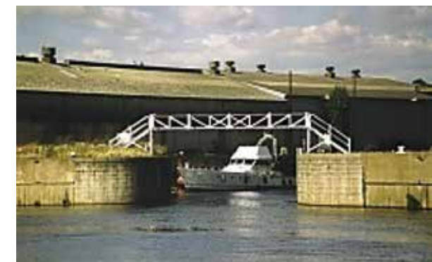
The old footbridge over the basin entrance as seen in Boon (Martin Underwood)
