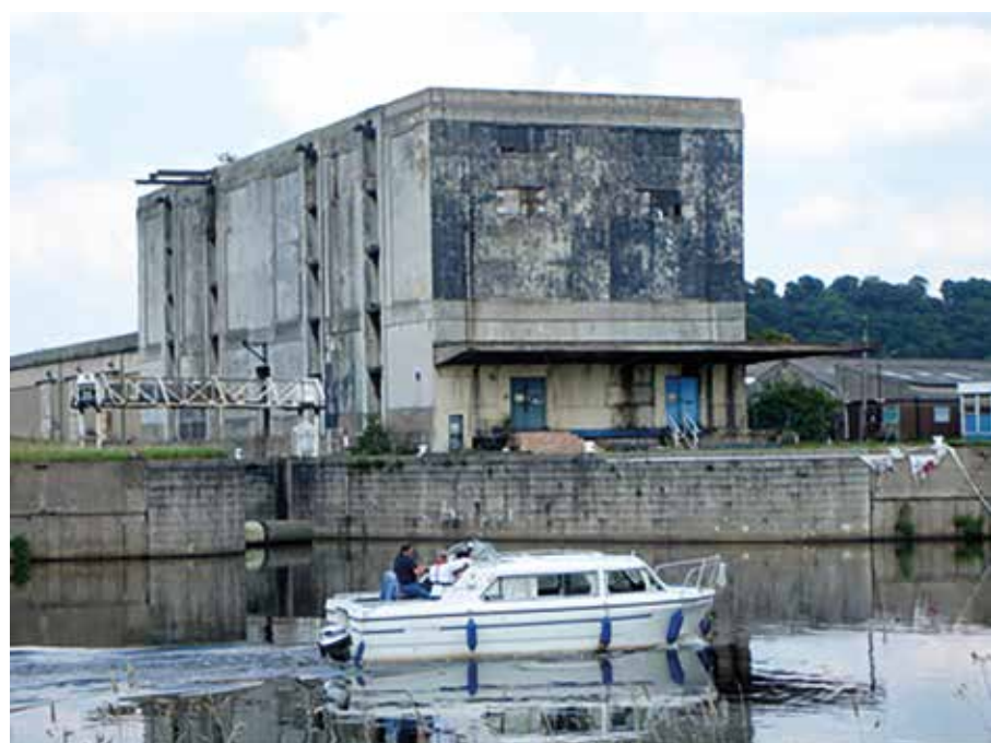
No.2 Warehouse not long before its clearance (Chris Matthews)
