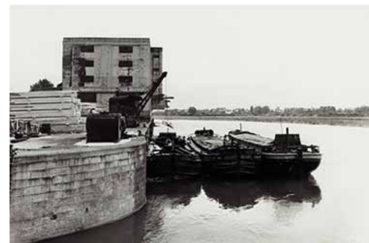
Here and in the picture below: cargo boats moored on opposite sides of the entrance to the basin.
