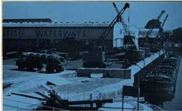
The wharf frontage at Meadow Lane Depot, Nottingham, with two of our Trent Fleet motor vessels alongside. Cuts of imported wire are being discharged on to our own berths for direct delivery to customers.
