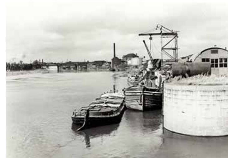
Lady Bay Bridge can be seen upstream (Canals & River Trust)
